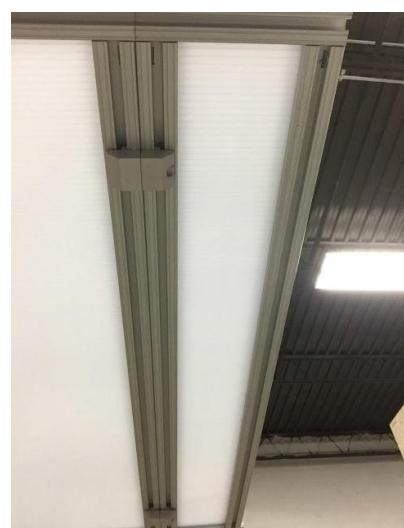
**✖ STEP SIX:** Slide the 5" door seal extension into the channel and tighten
