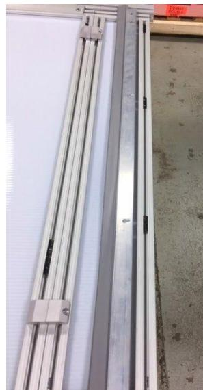
**✖ STEP EIGHT:** Reattach the threshold. The screws should still have the black, oval nuts in place. These slide into the channels on the underside of the door frame. Tight the screws.
