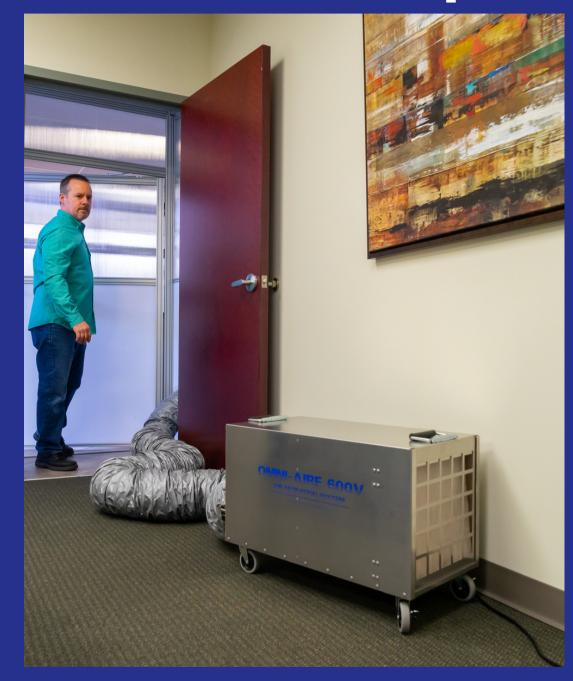
The air filtration system results in negative air pressure within the work enclosure space, further enhancing containment integrity.
