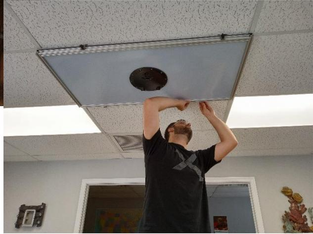
**Attach HEPA Filter and Ductwork**
